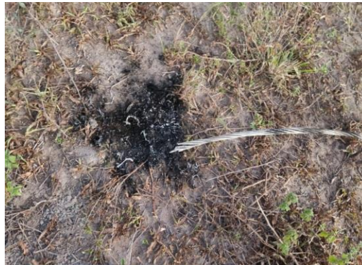
Figure 4 – Evidence of the arc formed when the cable touched the ground.
