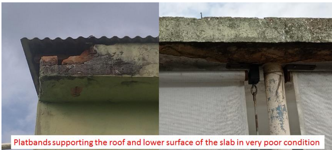
Figure 9 – Pathologies on the platbands and the underside of the slab in the external area. Source: Developed by the authors
